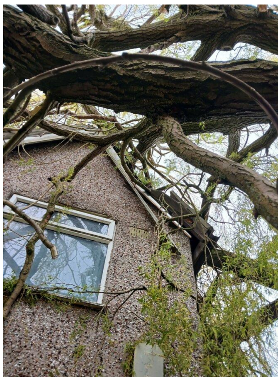
Figure 2: Large willow fell on to a house in Stainforth. Image: Rob Terrace
